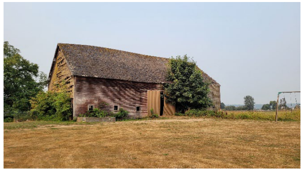
1887 Hanson Barn, 10632 99th Avenue SE
