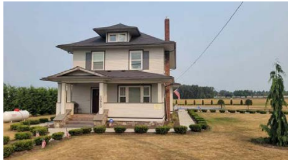
1931 Johnson Residence, 10520 Airport Way
