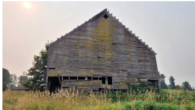
Northwest Elevations, Looking Southeast
