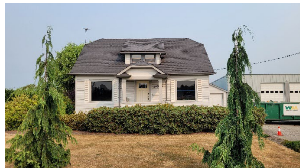
1931 Johnson Residence, 10530 Airport Way
